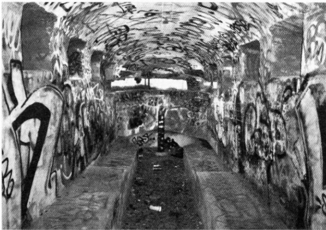
Pre-WWII gun emplacement, part of Stockholm's perimeter defences. Note the pintle mount for a heavy calibre quick fire (QF) gun at the end of the emplacement.
